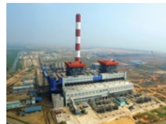
The 1,320-megawatt Sembcorp Gayatri Power facility in Andhra Pradesh, India
